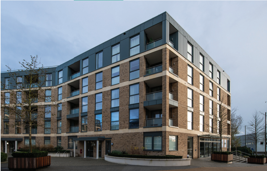
New purpose built premises and consultation rooms, Richmond Medical Practice, Kew, London. Owned and funded by PHP PLC.
