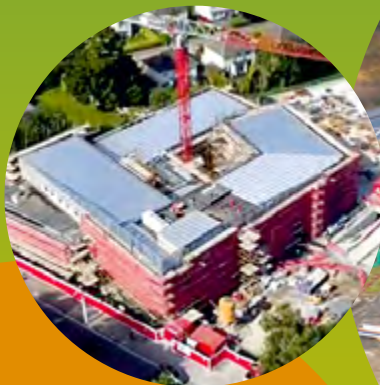
Bray Primary Care Centre, Wicklow, Ireland.
