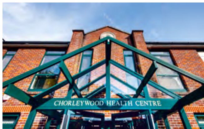
Chorleywood Health Centre, Rickmansworth, England.
