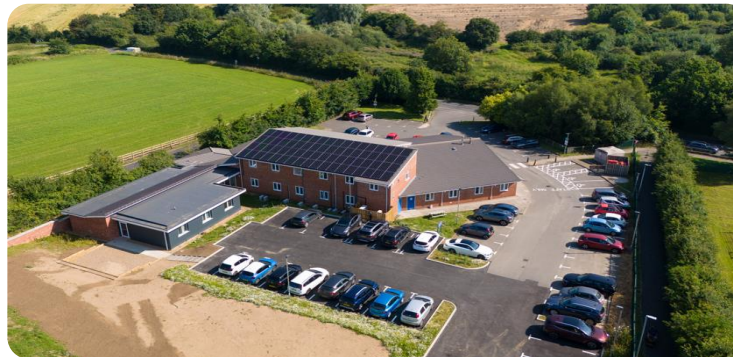
Long Stratton, Norfolk – PHP's first NZC asset management project
