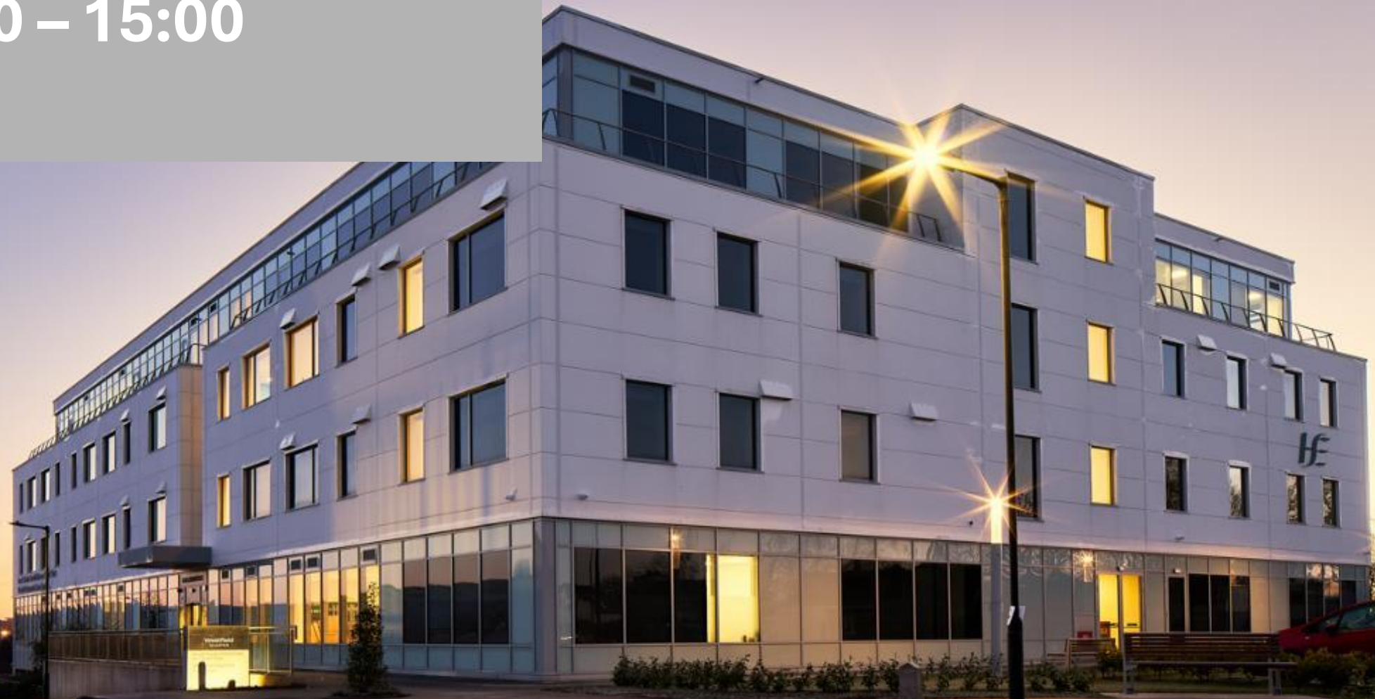
Westfield Integrated Primary Care Centre, Ballincollig
